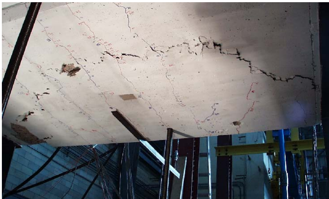
Figure 5-32: Exterior span failure at bottom of deck, facing south
