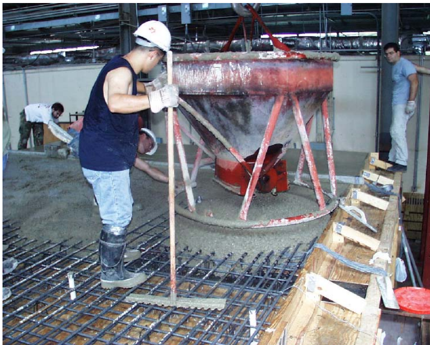
Figure 4-3: Placing concrete
