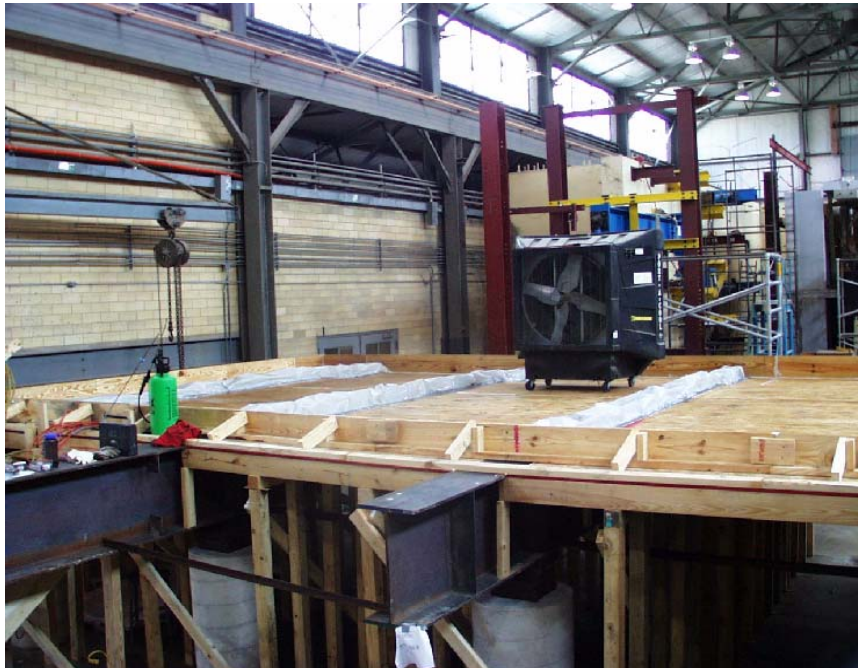
Figure 4-2: Finished formwork
