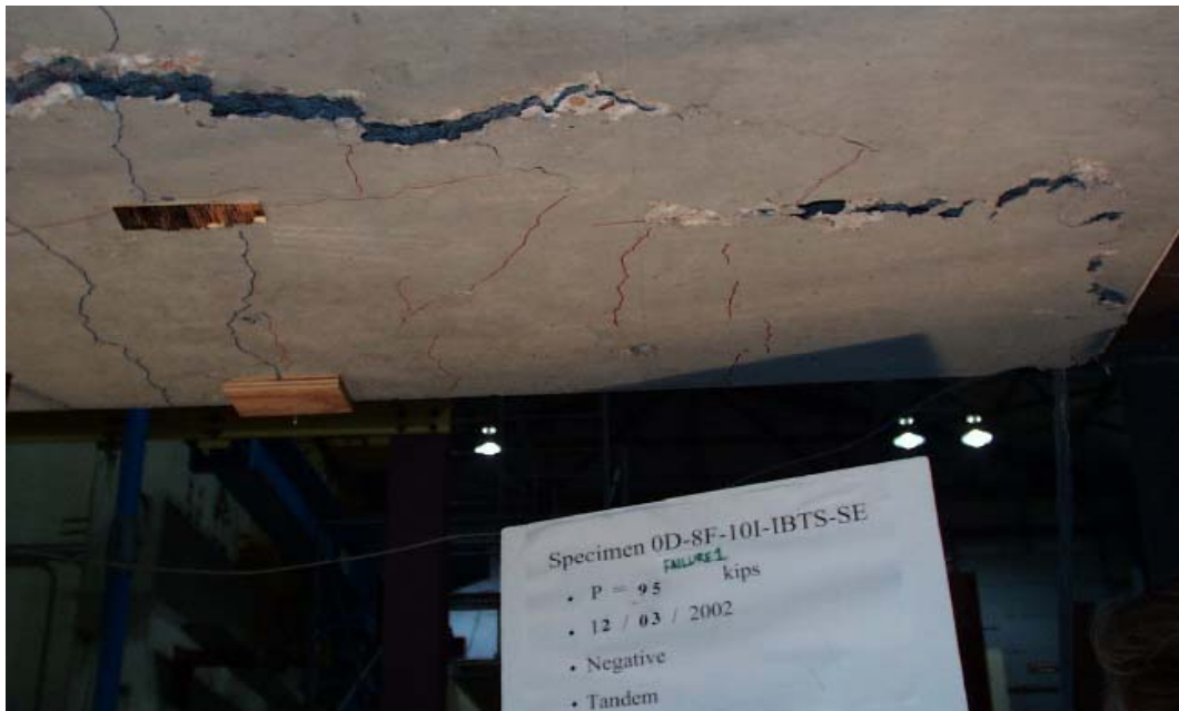
(ii) West side of interior span, facing south
