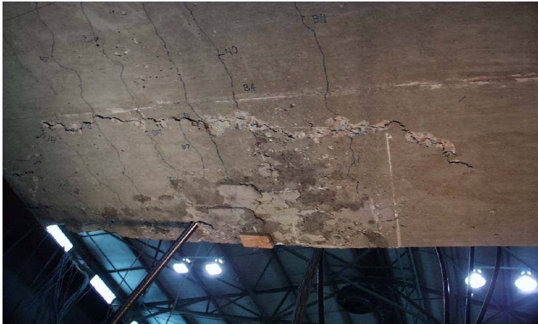
Figure 5-65: Exterior span failure at the bottom of the deck
