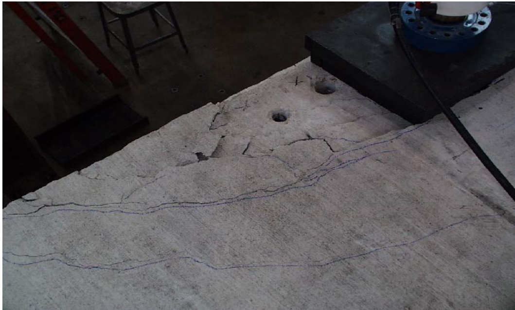
(i) East side of interior span, facing south
