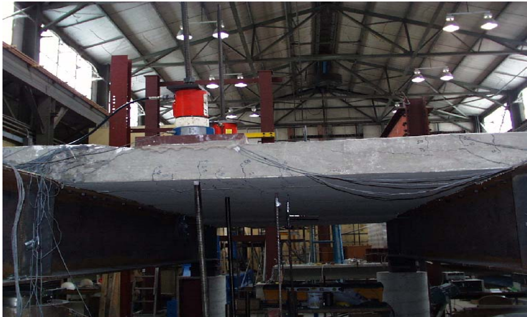
Figure 5-81: Interior span failure at side of deck, facing south
