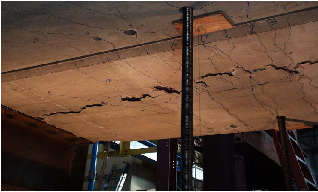
(i) East side of test span, facing south
