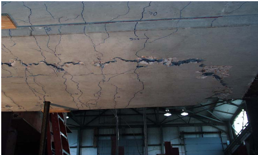
(ii) West side of test span, facing south
