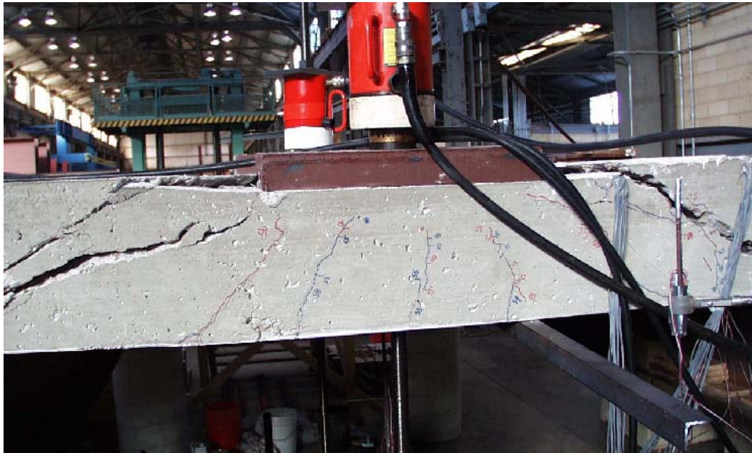
Figure 5-33: Exterior span failure at side of deck, facing north
