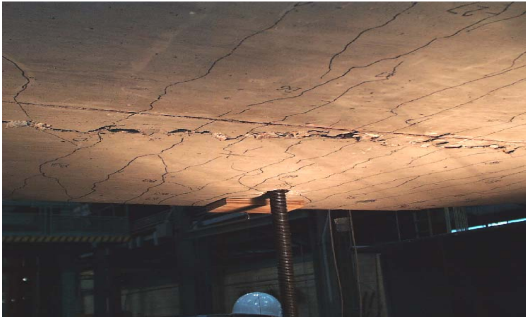
Figure 5-54: Northwest test area failure at bottom of deck, facing north
