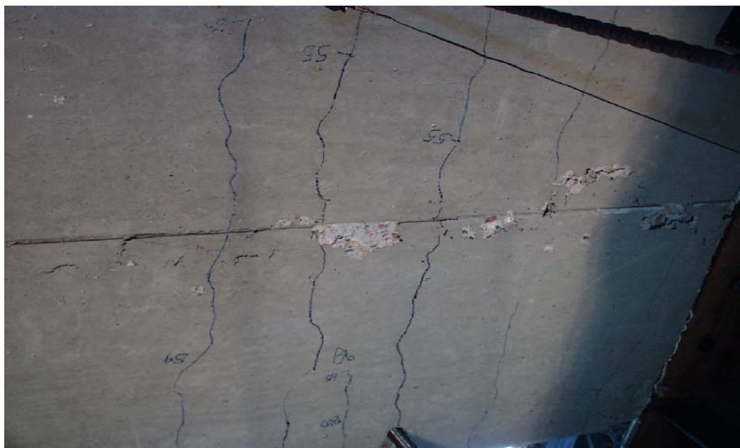
Figure 5-80: Interior span failure at bottom of deck, facing south
