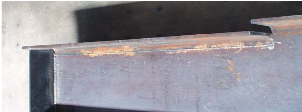
Figure 4-1: Girder flange drop down
