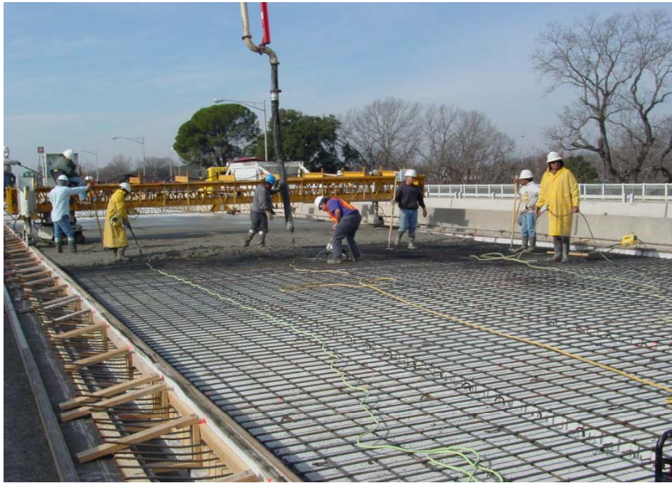
Figure 1-6: Placing of concrete in the field
