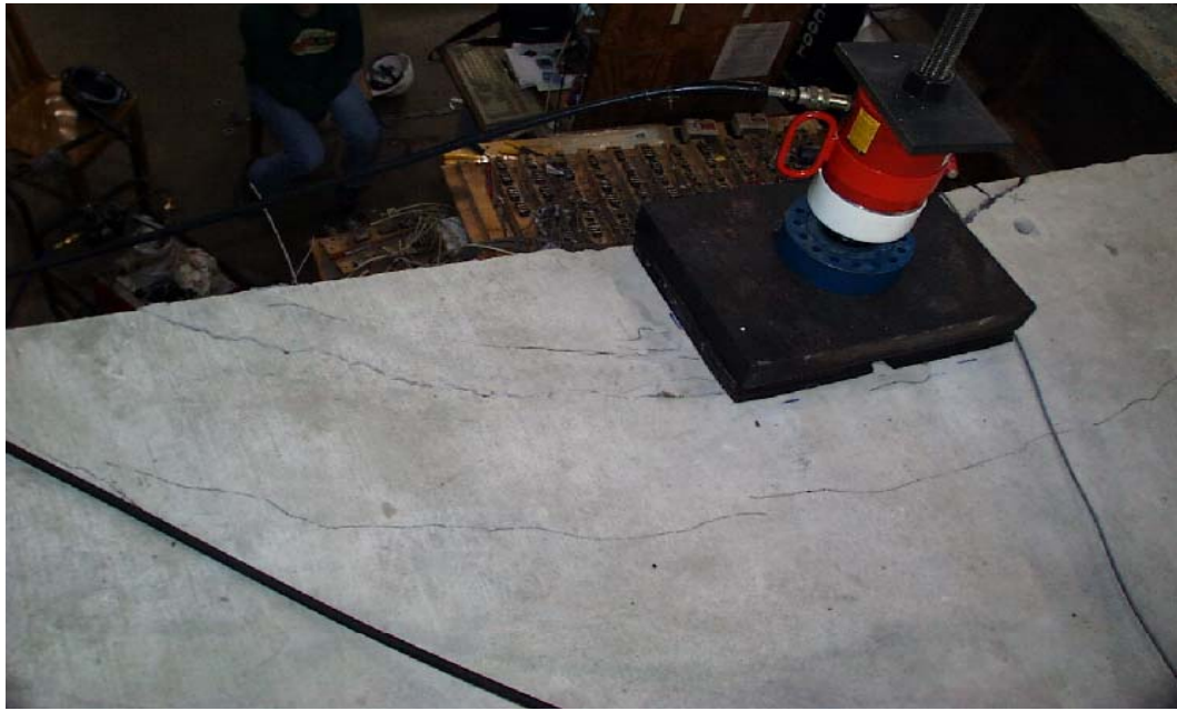
Figure 5-56: Northwest test area failure at top of deck, facing north
